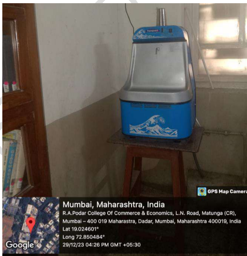
Plate 9: Drinking water facility in the premises
